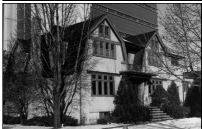
Top: Front view of the Divine Temple Church of God. Middle: The church interior reveals elaborate woodwork drawn from English Gothic precedents and is noted for its open roof design. Bottom: Fannie D. Johannes Memorial Hall, built in 1924. Photos used with permission, courtesy of the Wisconsin Historical Society.
